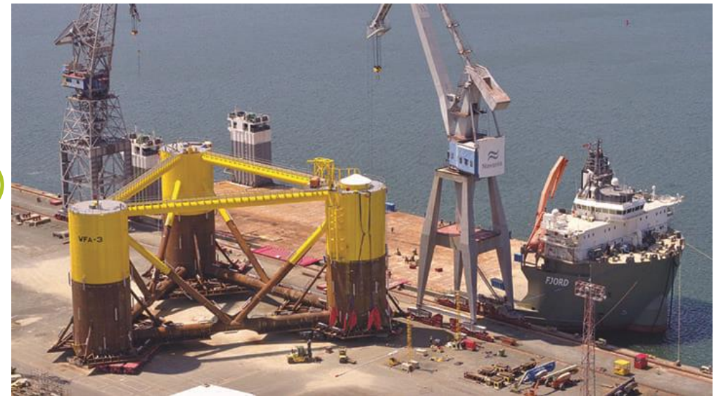
A “WindFloat” semi-submersible substructure at port. At present, only a few ports globally can handle the scale of these structures.
