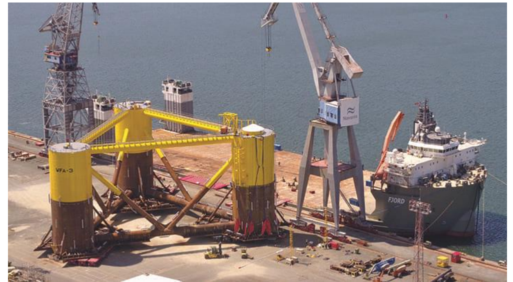
A "WindFloat" semi-submersible substructure at port. At present, only a few ports globally can handle the scale of these structures.
